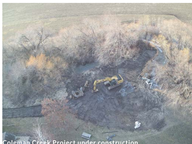
Coleman Creek Project under construction
